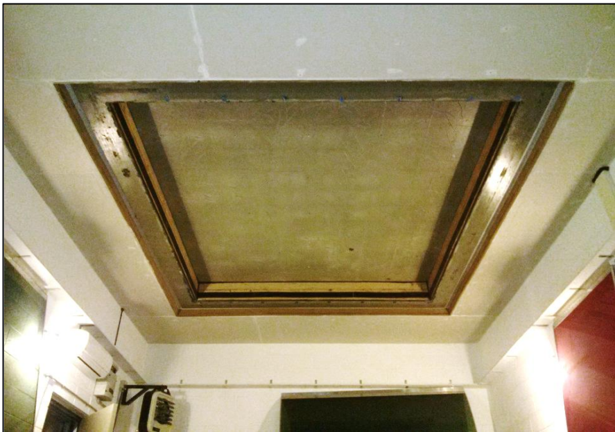
Receive Room View of Test Specimen Installation
